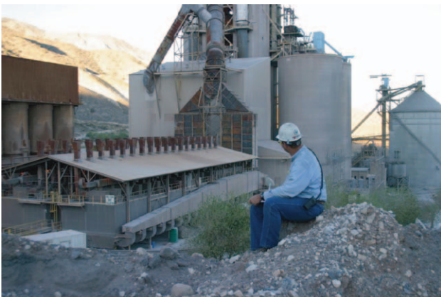
Figure 2. Main reverse air kiln baghouse.
